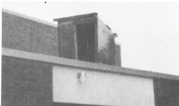
The ultimate in restrooms.
